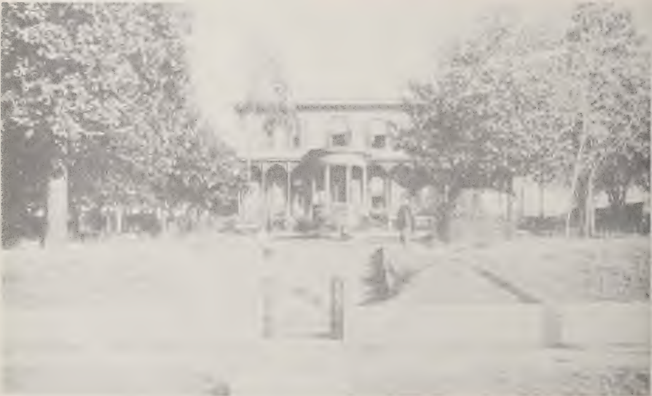
Vincentelli-Nicrosi home on Jackson Street at the head of Washington Avenue has been demolished. (1890)
